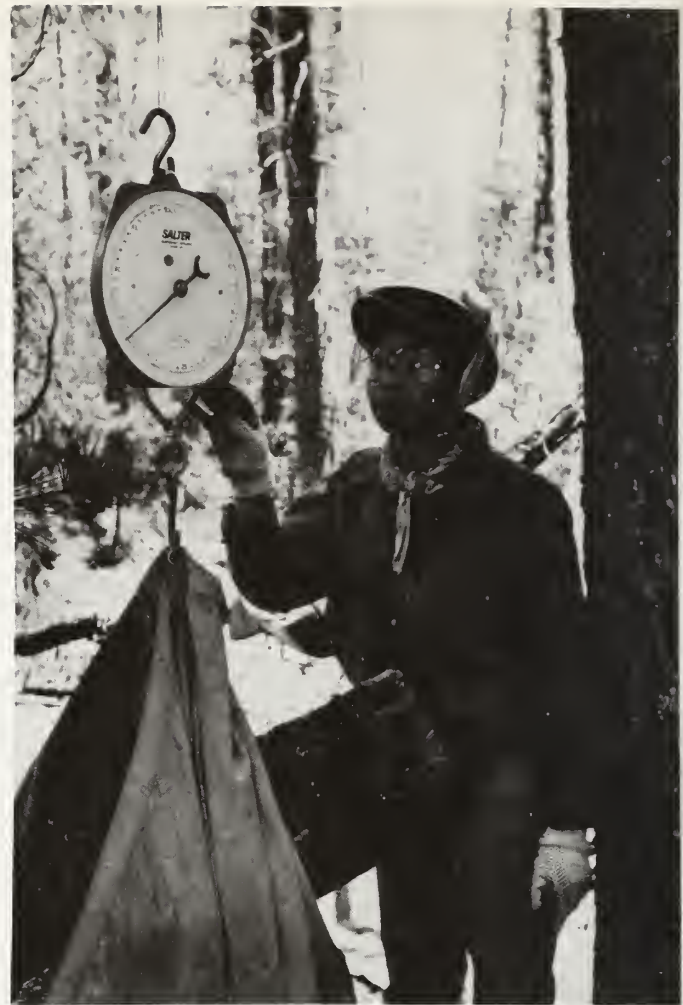
Weighing lodgepole pine bole sections to determine volumes of useable material.
